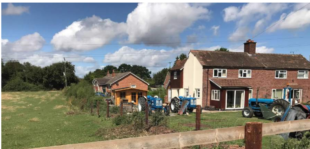
Figure 7. Existing development at Castle Park, Kilpeck.
